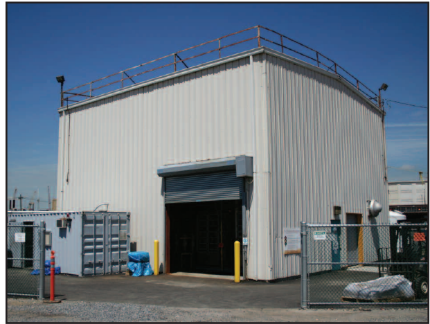
Water Treatment System
